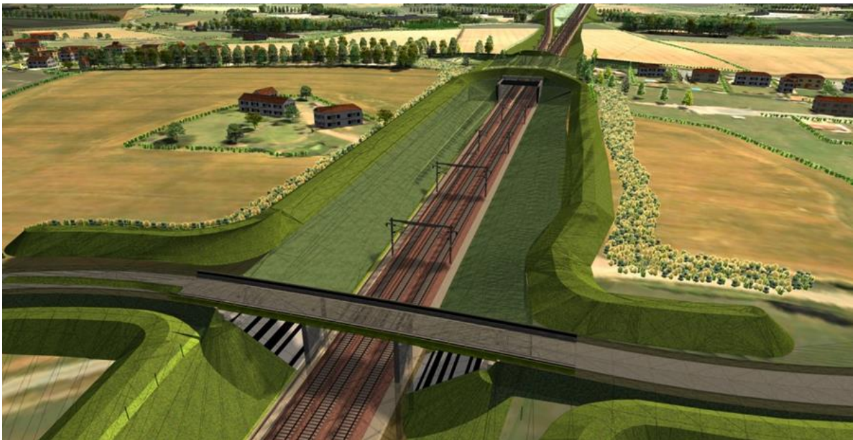
Perspective view of a railway crossed by a road and wildlife bridges
